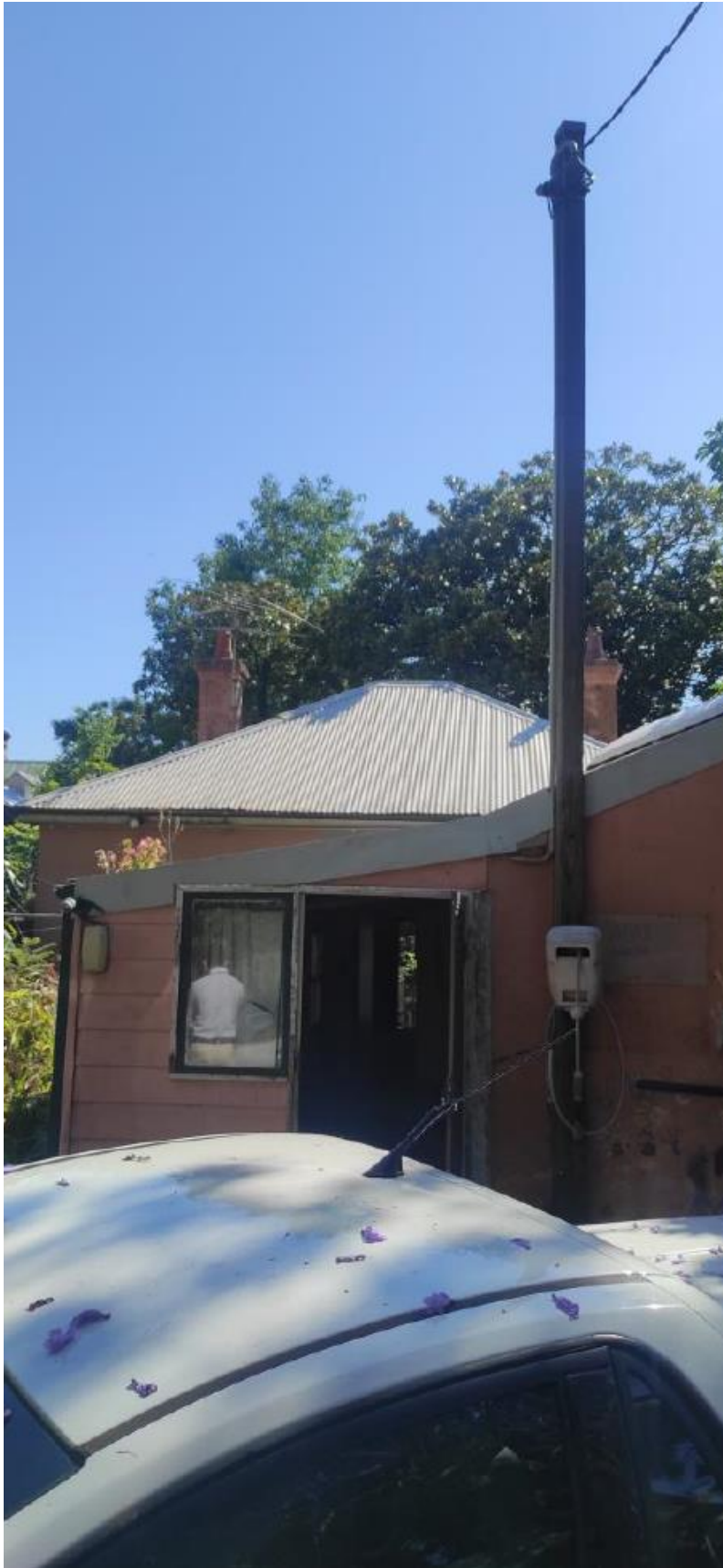
Figure 10: Rear elevation of property viewed from rear yard
