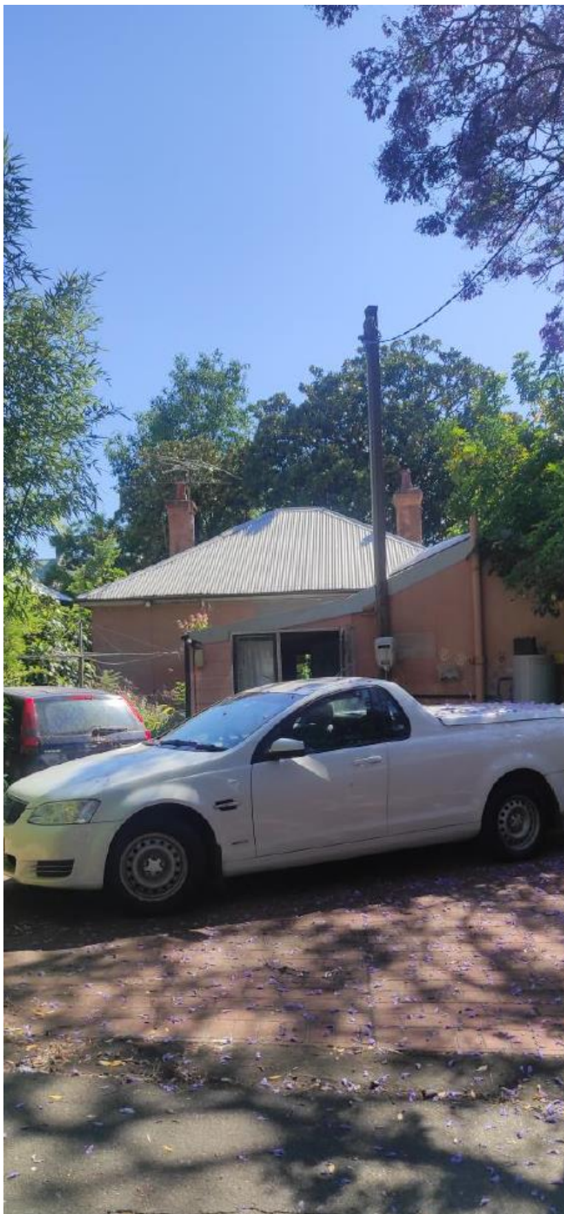
Figure 12: Rear elevation of subject site as viewed from Derwent Lane
