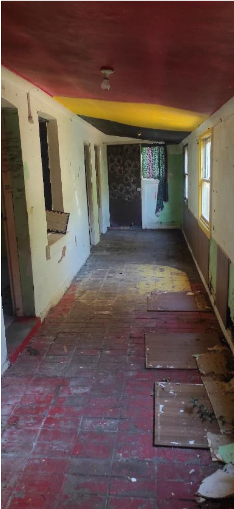
Figure 9: Internal photo of existing rear addition (to be demolished)
