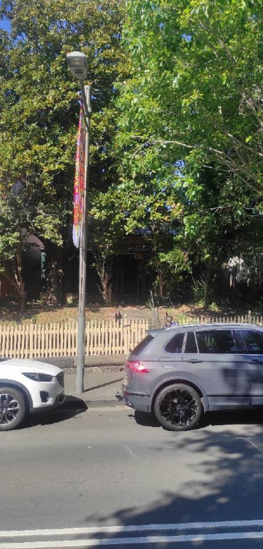
Figure 2: Front elevation of subject site viewed from Glebe Point Road
