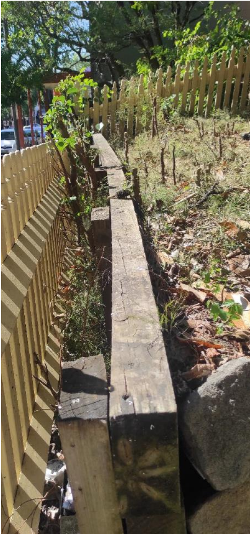
Figure 5: Existing retaining wall on Glebe Point Road frontage
