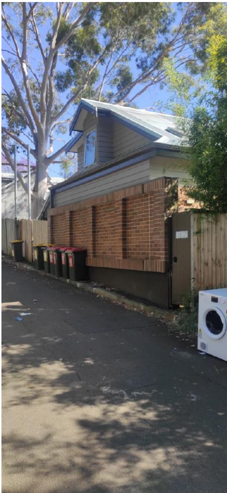
Figure 13: Rear of neighbouring property at No. 122 Glebe Point Road as viewed from Derwent Lane
