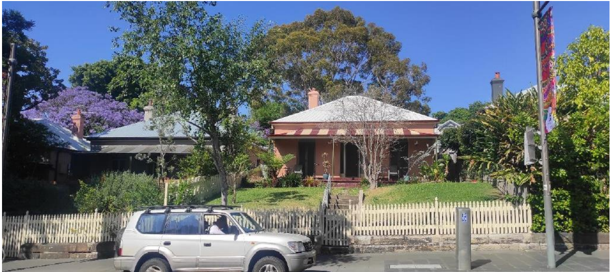
Figure 4: No. 124 Glebe Point Road (Part of heritage terrace group).
