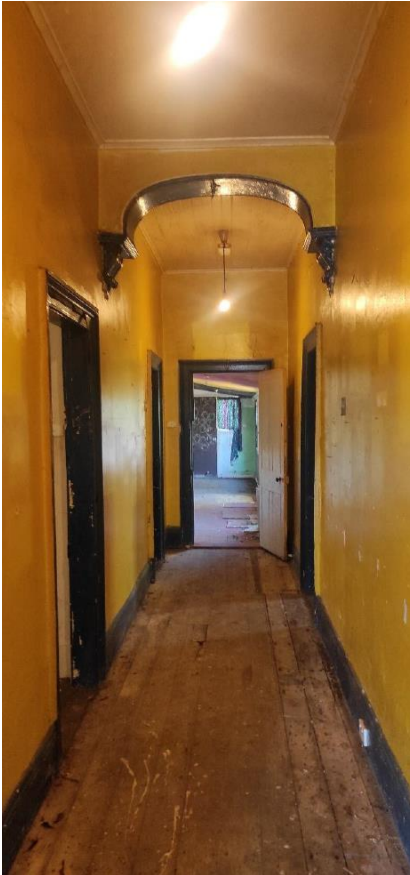
Figure 8: Internal photo of main hallway (main building)
